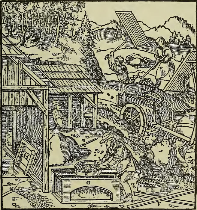
A—SCREEN. B—POLES. C—SHOVEL. D—TWO-WHEELED CART. E—HAND-SIEVE. F—NARROW BOARDS. G—BOX. H—COVERED PIT
