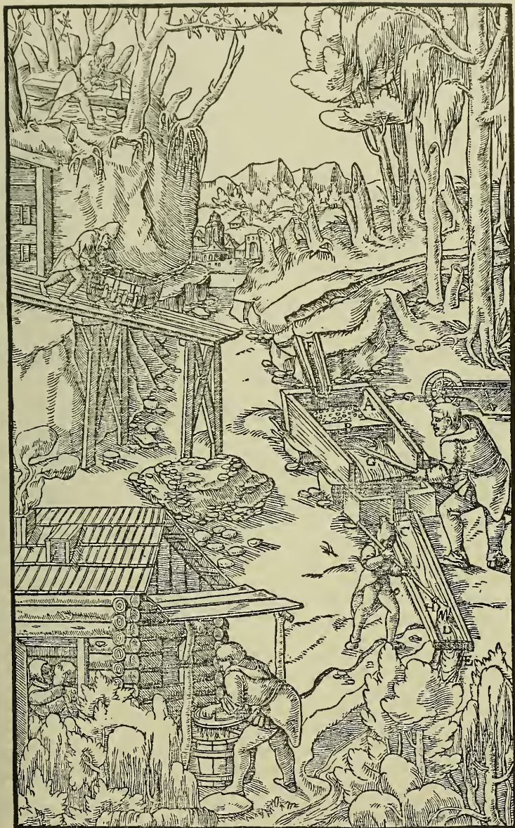
A—BOX. B—PERFORATED PLATE. C—TROUGH. D—CROSS-BOARDS. E—POOL. F—LAUNDER. G—SHOVEL. H—RAKE.
