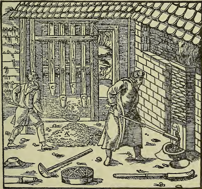
A—CHARCOAL. B—MORTAR-BOX. C—STAMPS.
