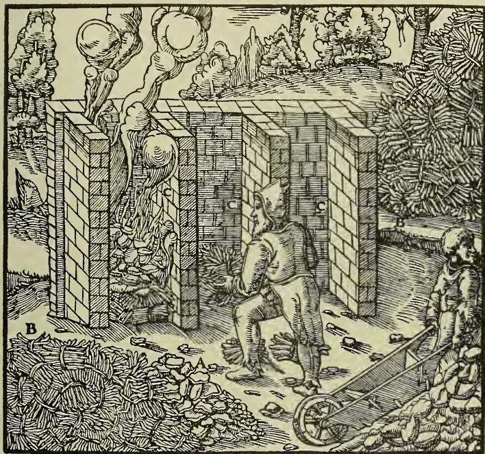
A—CAKES. B—BUNDLES OF FAGGOTS. C—FURNACES.
