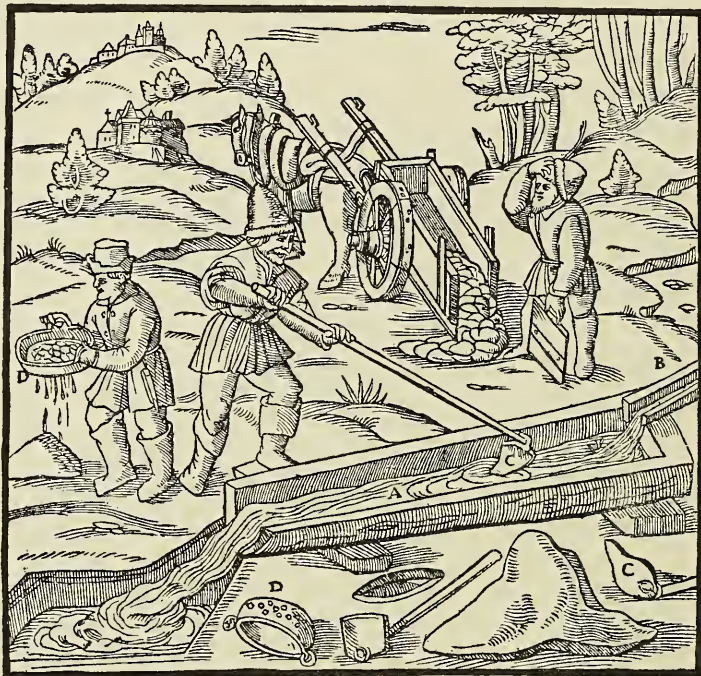
A—TROUGH. B—LAUNDER. C—HOE. D—SIEVE.
