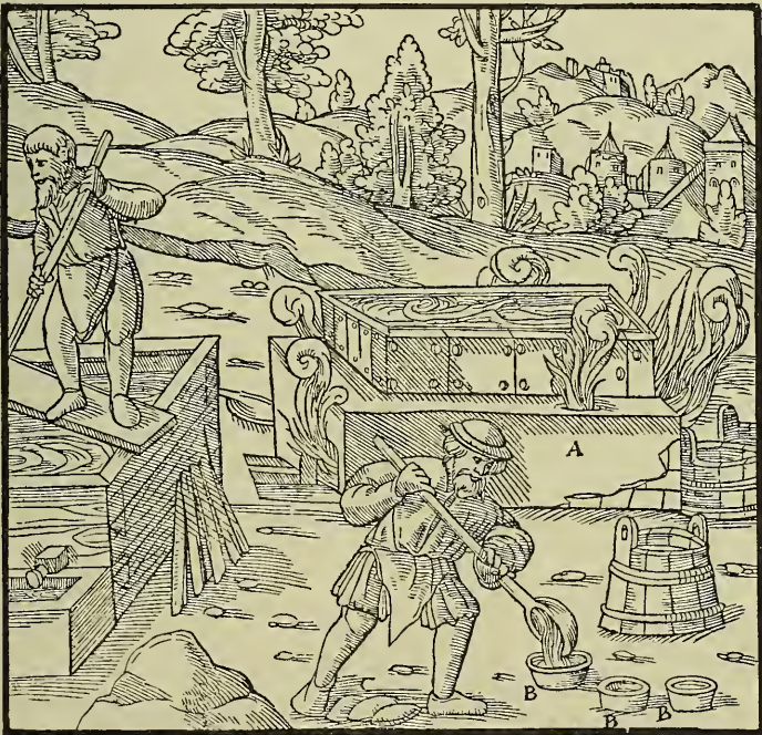
A—CALDRON. B—MOULDS. C—CAKES
