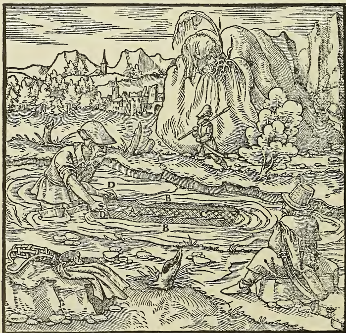
A—PLANK. B—SIDE-BOARDS. C—IRON WIRE. D—HANDLES.
