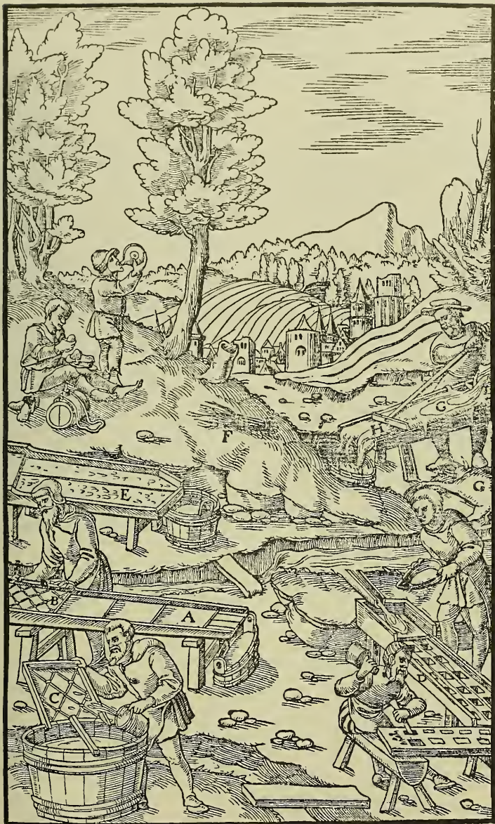
A—SLUCE COVERED WITH CANVAS. B—ITS HEAD FULL OF POCKETS AND GROOVES. C—HEAD REMOVED AND WASHED IN A TUB. D—SLUCE WHICH HAS SQUARE POCKETS. E—SLUCE TO WHOSE PLANKS SMALL SHAVINGS CLING. F—BROOM. G—SKINS OF OXEN. H—WOODEN SCRUBBER.
