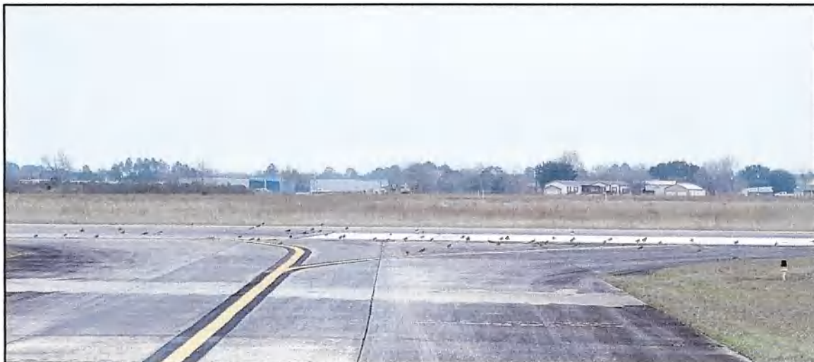
Figure 4. Example of wildlife hazard. (Photo provided by the Airport.)
