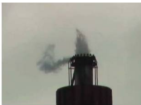
Poorly Operating Flare/Over Steamed – Low Combustion Efficiency
