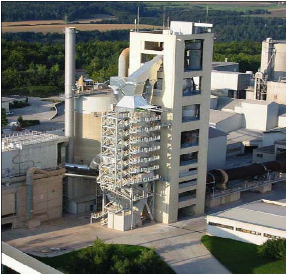
Figure 4-1.1 SCR on Preheater Tower at Solnhofen Zement, Germany
