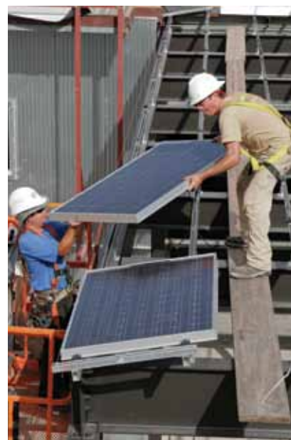
Solar panel installation at the Pearl Brewery
