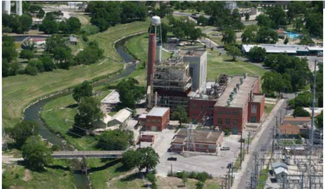
Mission Road Power Plant
