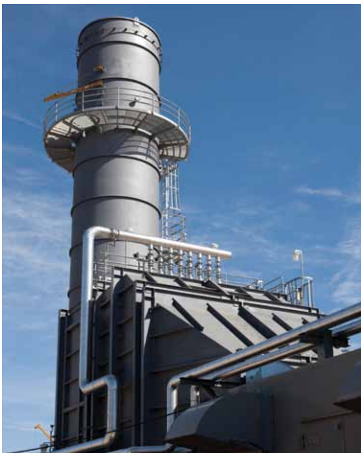
Braunig peaking units under construction
