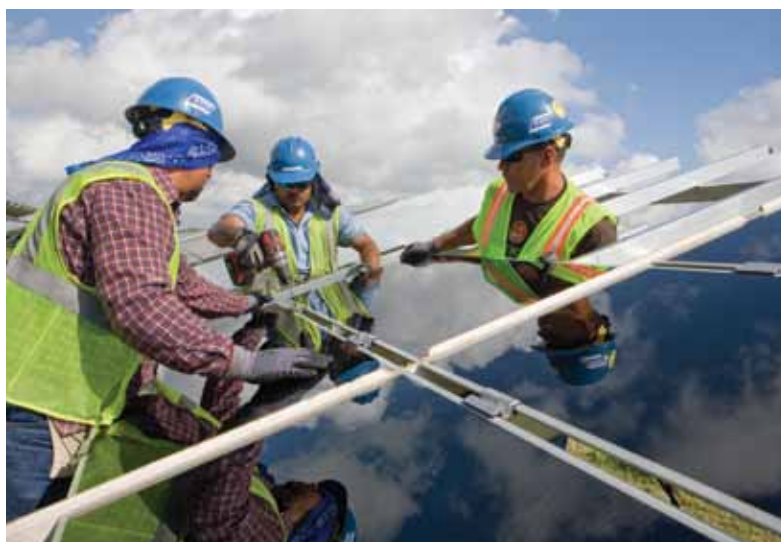
Blue Wing Solar Project under construction
