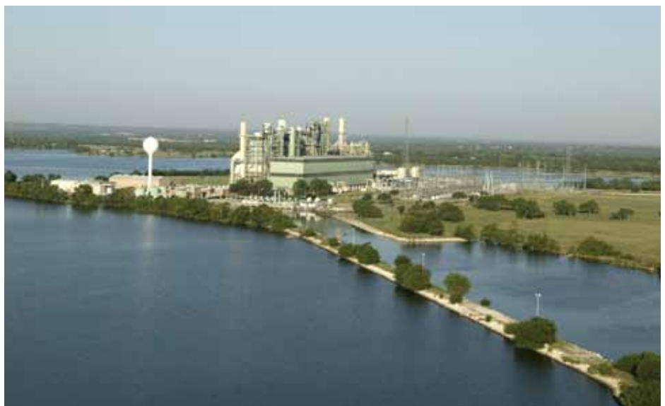
Braunig Power Station
