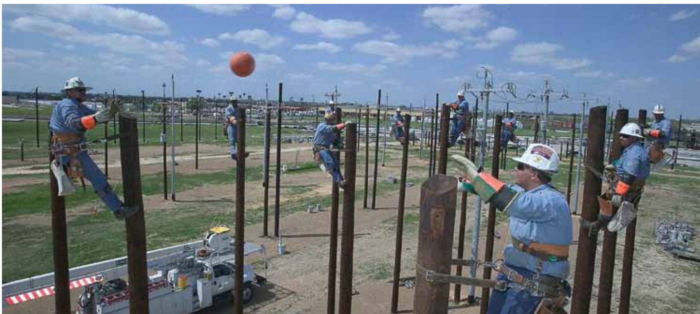
Linemen training at the Southwest Service District
