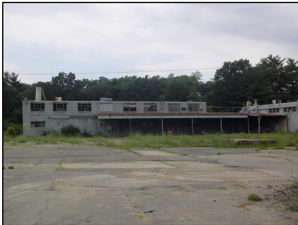
View of one of the existing building which will be demolished
