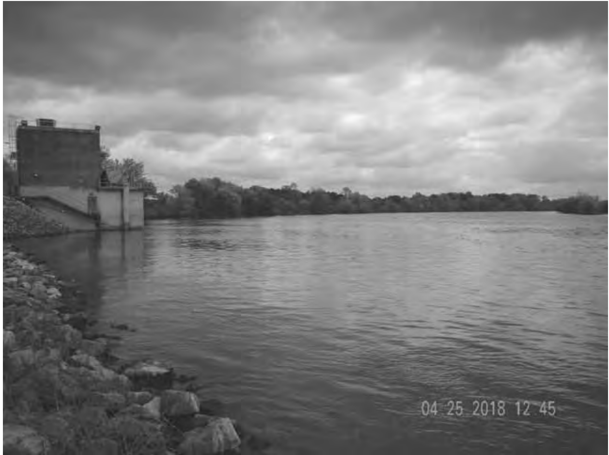
Figure 5: GI00 Upstream View
