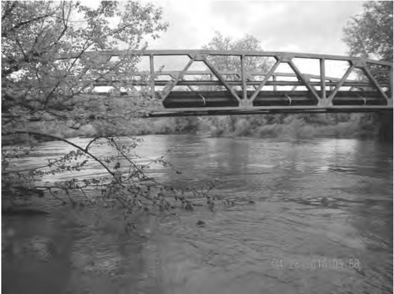
Figure 20: CT04 Upstream View
