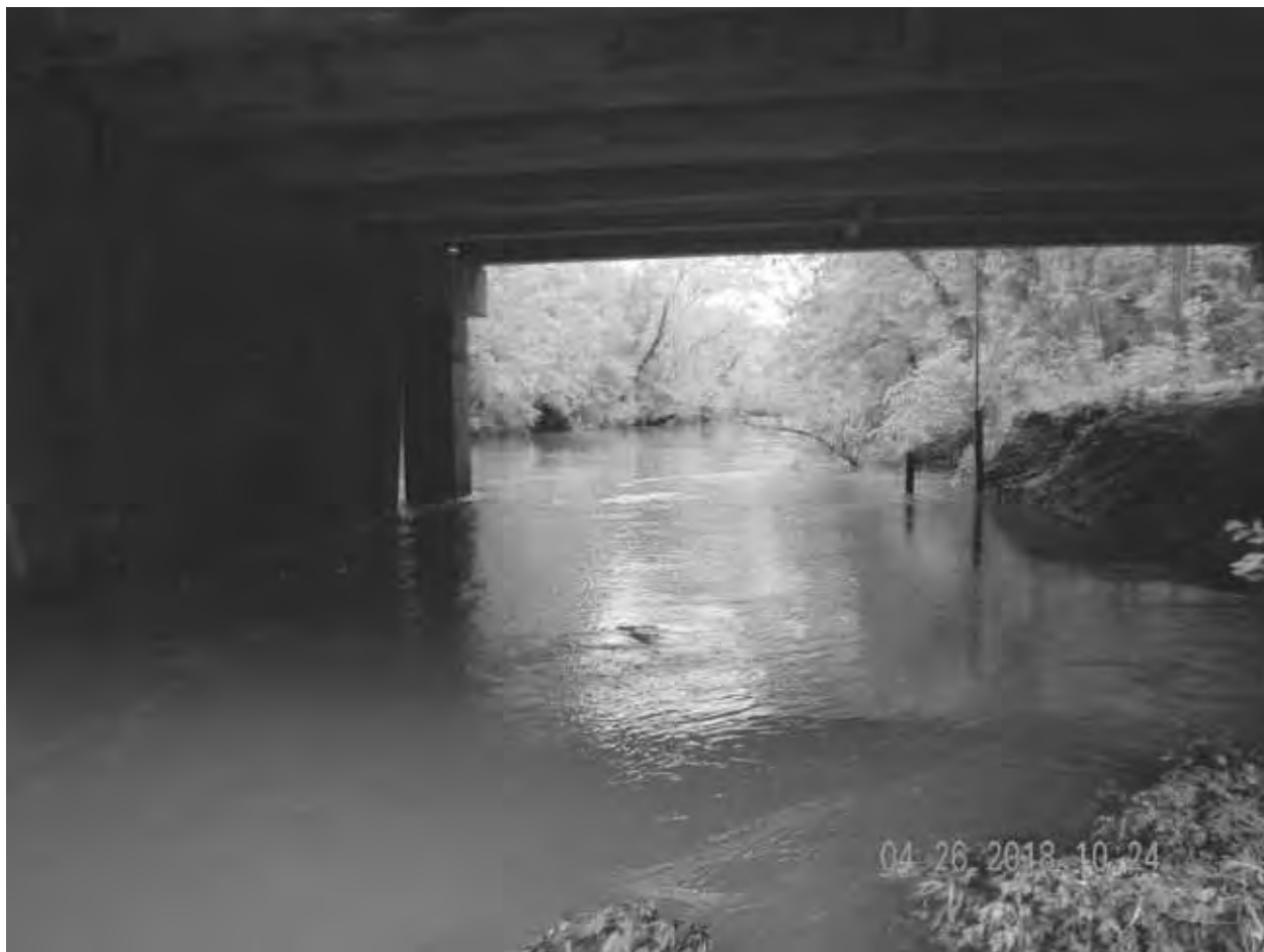
Figure 22: CT05 Upstream View
