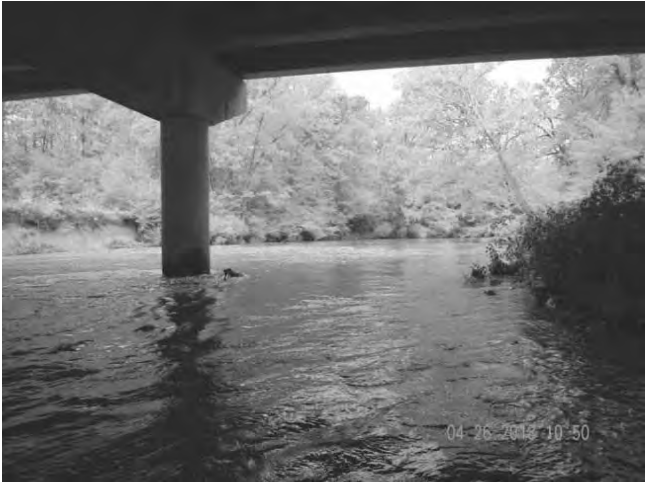
Figure 24: CT05 Upstream View
