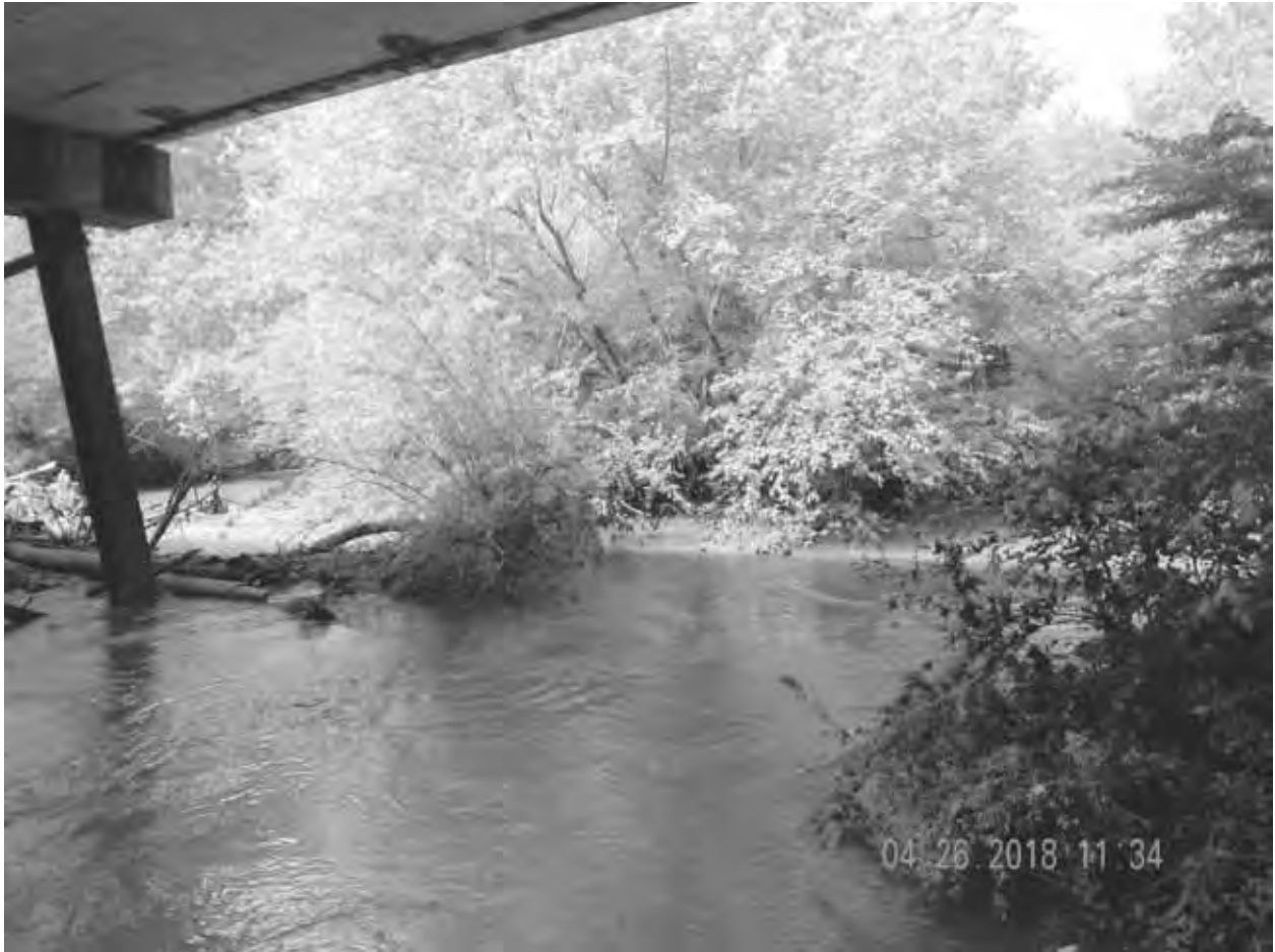
Figure 29: CT08 Upstream View
