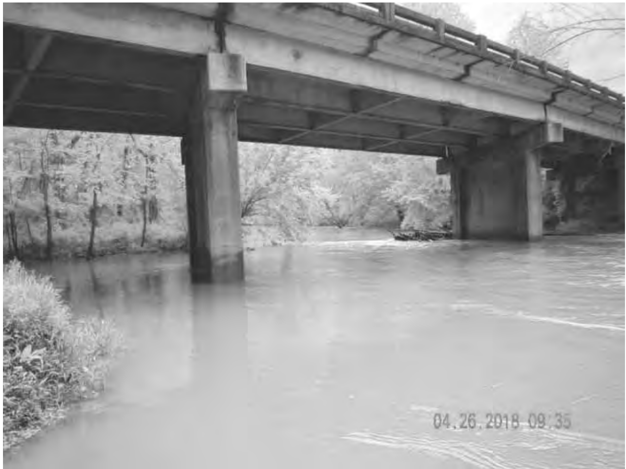
Figure 18: CT03 Upstream View
