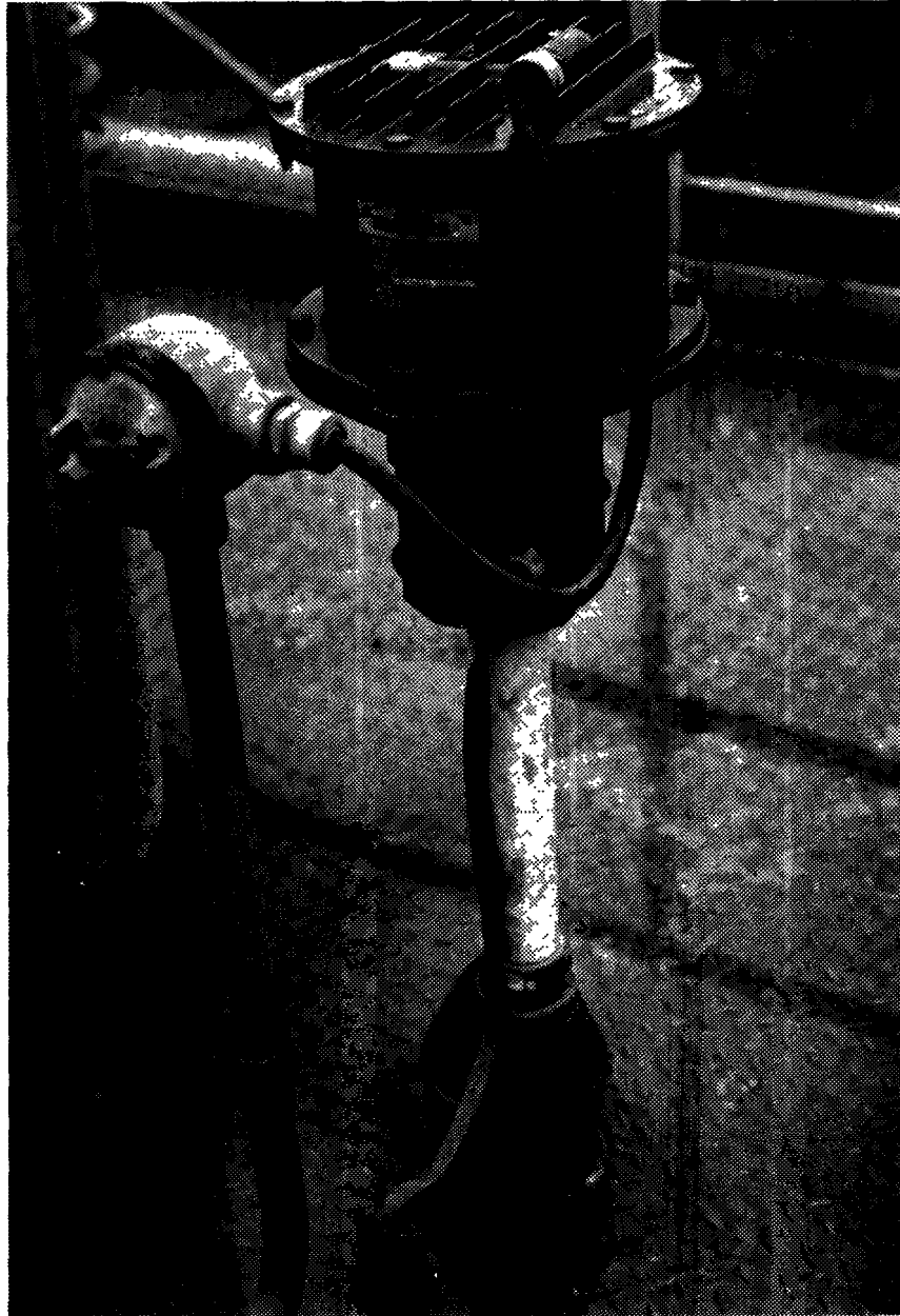
Figure 2-20. Typical electric vibrator type rapper.
