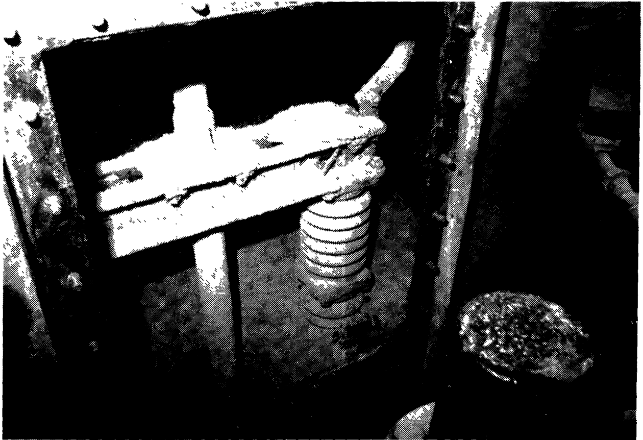
Figure 6-19. Insulator compartment showing dust deposits.
