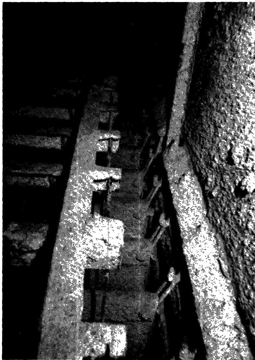
Figure 6-13. Upper baffle used as plate suspension.
