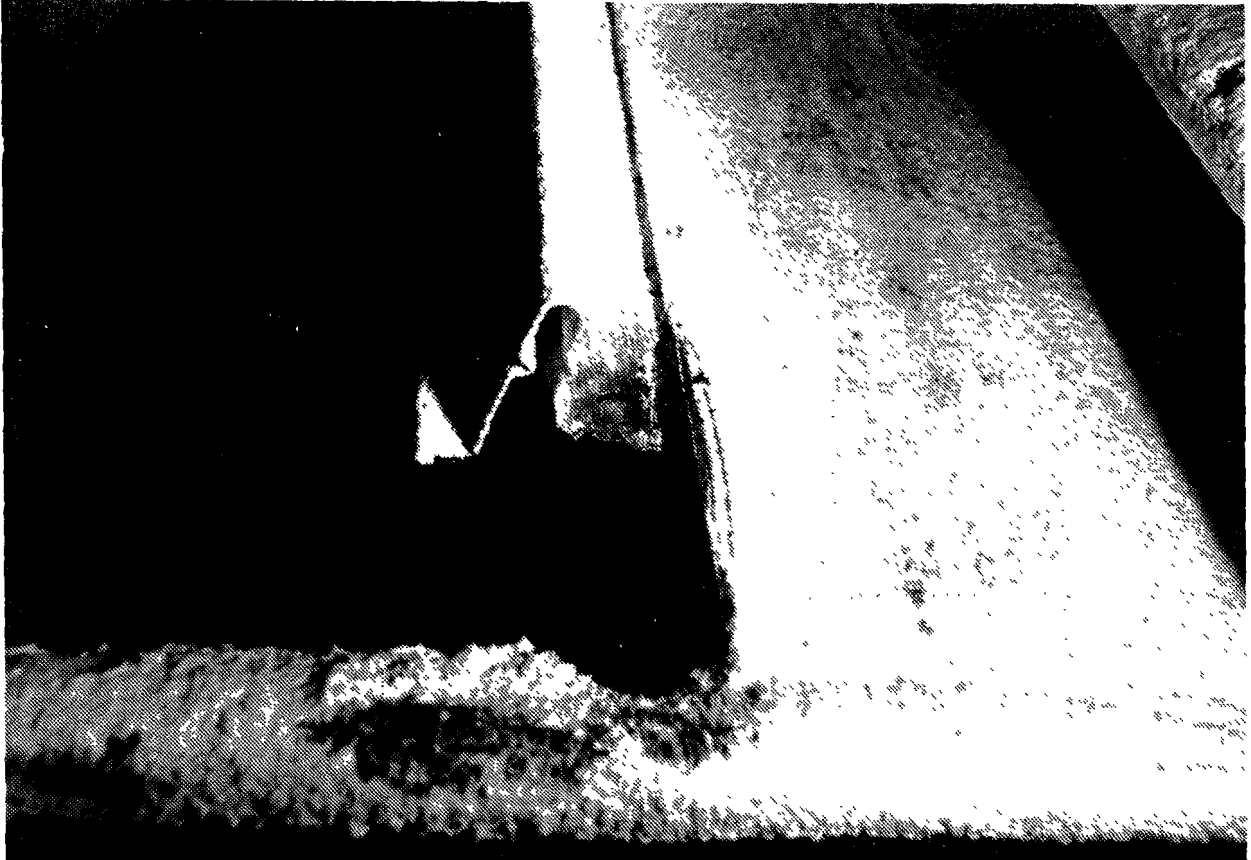
Figure 6-20. Example of plate cracks.
