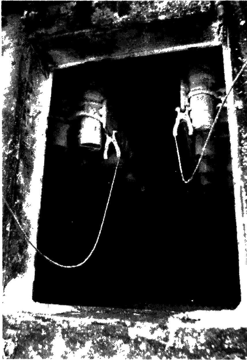
Figure 7-3. Ground clips.
