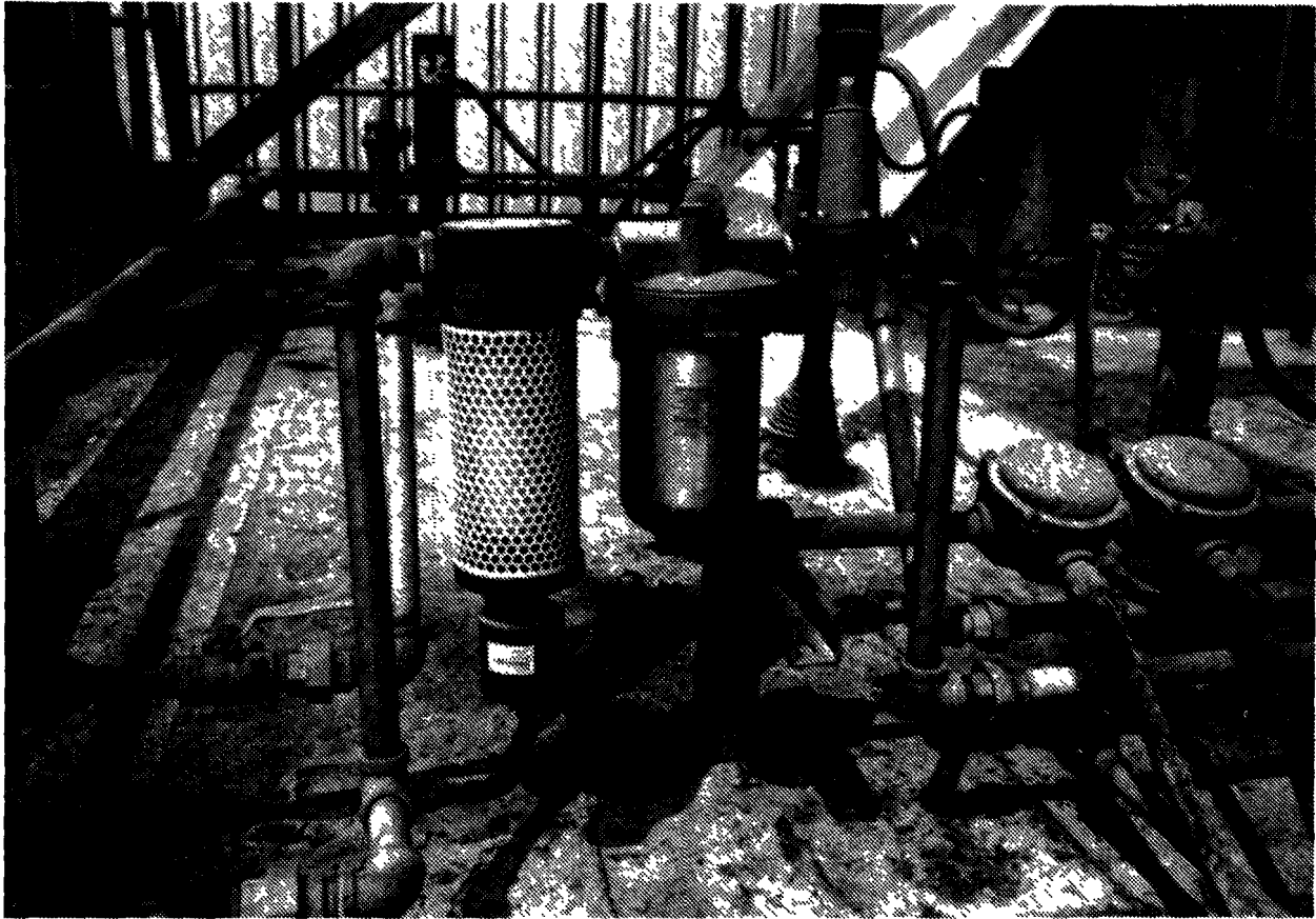
Figure 6-1. Rapper air line trap and filter.
