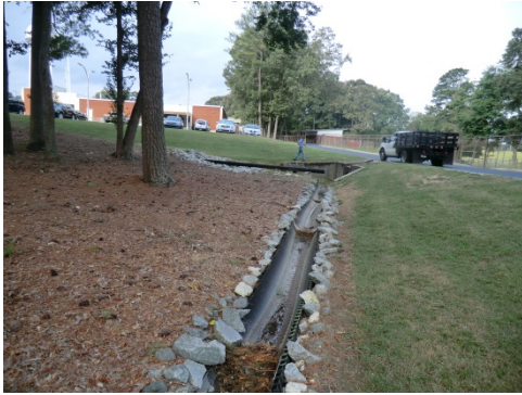
Stream 1 – Ephemeral segment, facing downstream (west) from origin of channel.
