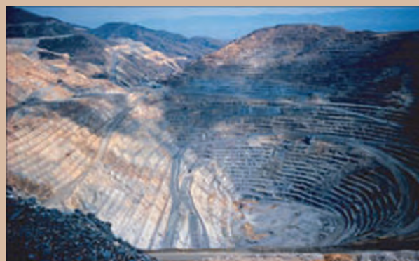
Visible from space, the Bingham Canyon copper mine in Utah has produced more than 12 million tons of porphyry copper. The mine is more than 4 kilometers (2.5 miles) across at the top and 800 meters (0.5 mile) deep and is one of the engineering wonders of the world. Photograph by C.G. Cunningham, USGS.
